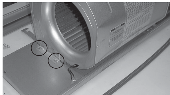
Figure 17 – Disconnect Blower Housing
