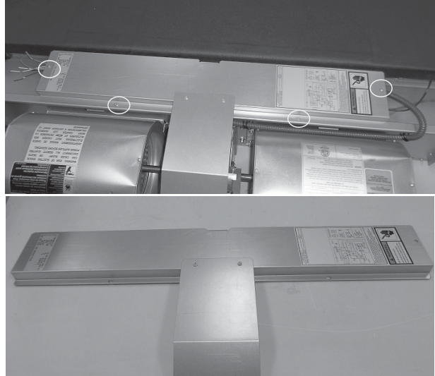
Figure 7 – Control Box Cover Removal
