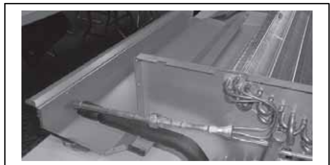
Figure 24 – Remove Condensate Baffle Assembly
