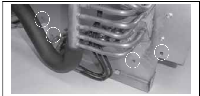
Figure 23 – Condensate Baffle Screws
