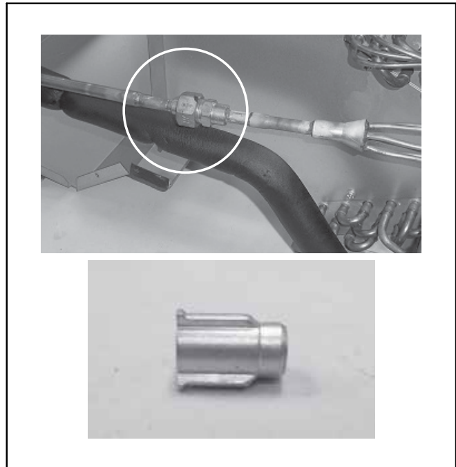
Figure 25 – Metering Device Location / Piston (FMC4P, FMU4P, WAMC Units)
