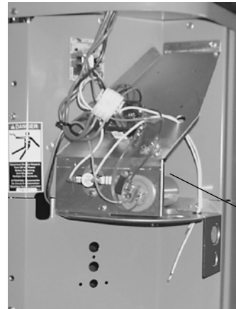
Outdoor Temp. Sensor Location in Outdoor Unit Typical Mounting
