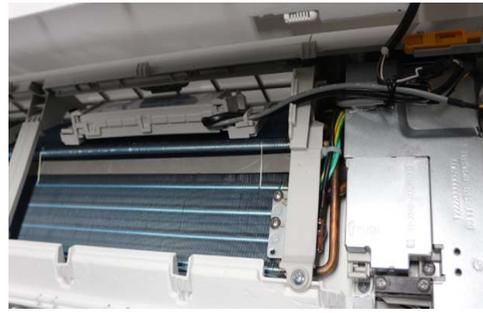
**Fig. 33 — Use ties to keep wiring aligned**
