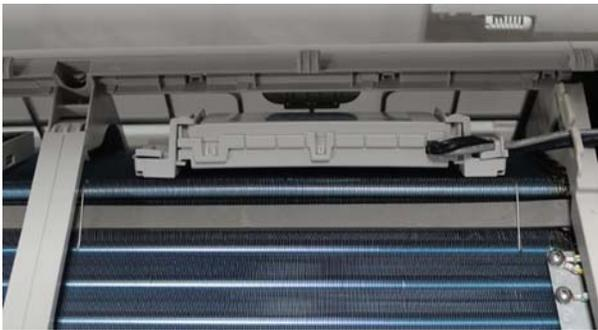
**Fig. 31 — Install the multi-function board**
