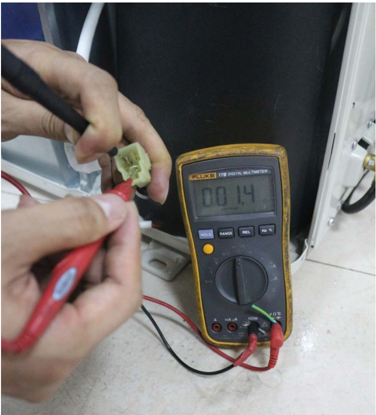
Fig. 61 – Test the voltage
